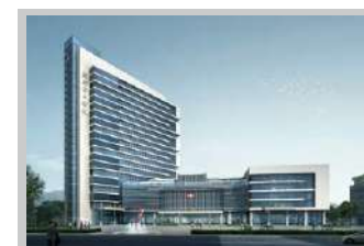
Hospital sewage treatment
