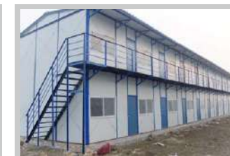
Temporary construction site sewage
